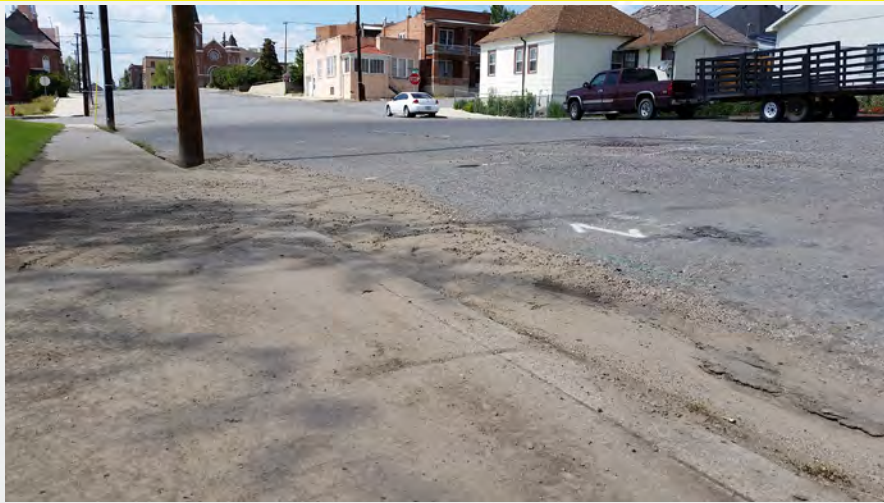
Sediment clogging a gutter after a thunderstorm Photo Dave Hutchins
