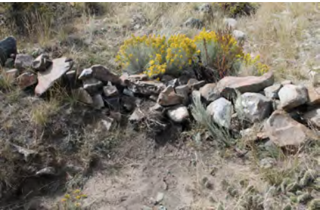
Sediment and debris that has built up behind one of the rock weirs
